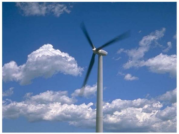
The QDLM V80-2.0 MW turbine is a pitch- regulated turbine with three blades and an 80metre rotor diameter. The revolution speed of the rotor varies between 9 and 19 rpm, and it is this flexibility that makes it ideal for placement in areas with modest wind speeds.
