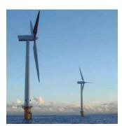
There are two versions of the V66 turbine: a 2.0 MW model for offshore sites, and a 1.75 MW model for inland locations. Both versions feature a rotor diameter of 66 meters, hub heights of 60—78 meters, and, last
