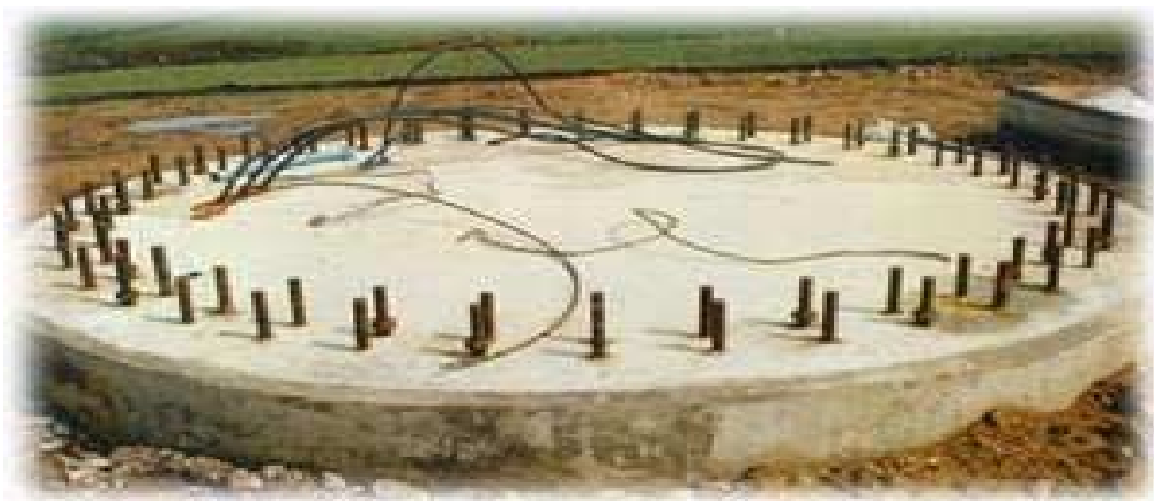
3. Wind farm substructure - Ghana, West Africa
