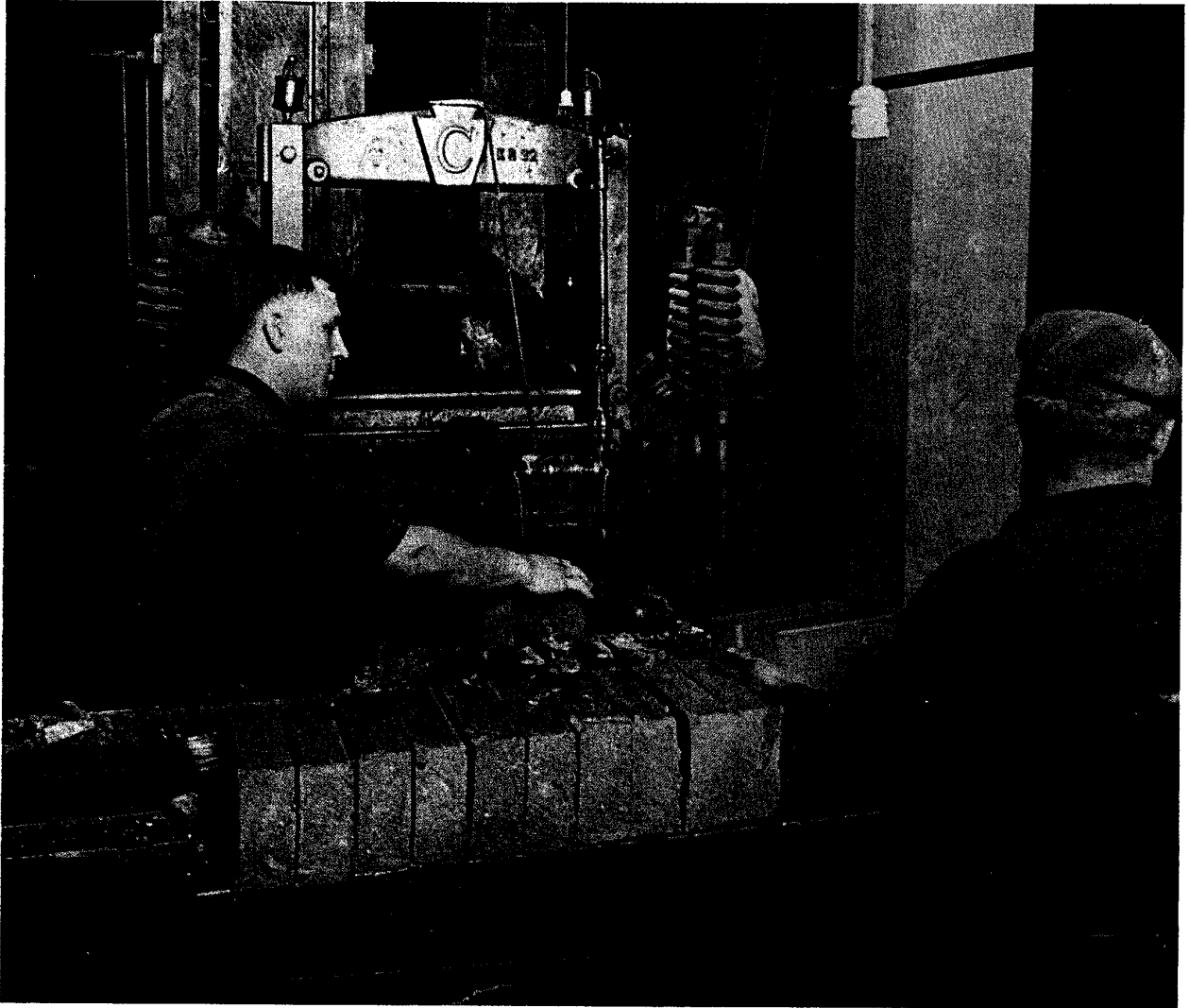
In the young nation construction was a booming business. Particularly in cities, brick was a choice building material, since it is strong, easy to manipulate, and, above all, fire resistant. Courtesy Hagley Museum and Library.
